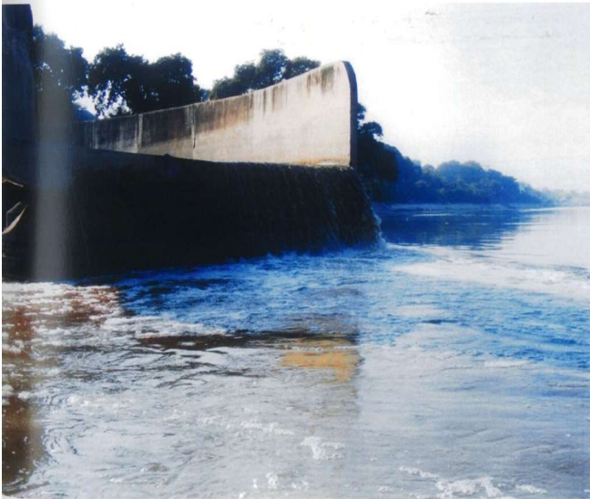
Power House Nala (main) - Near Parmath (Behind Elgin Mill)
