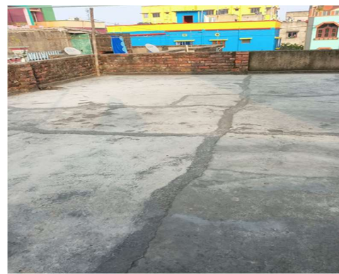
Figure – 11: Final Result after crack mending
