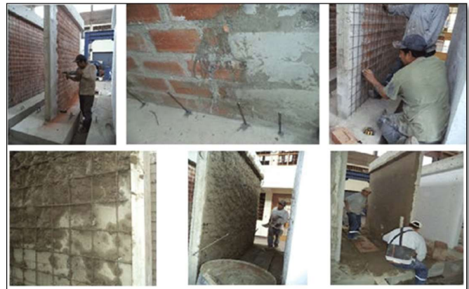
Figure – 4: Retro Fitting work at Site
