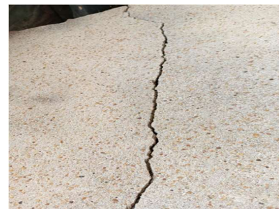
Figure – 4: Cracked Brick Wall
