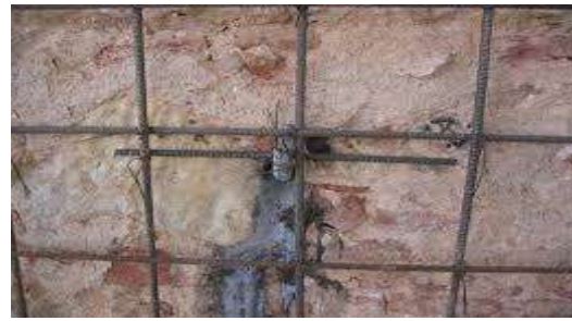
Figure - 3: Application of Steel Bars in old wall restoration
