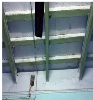
Figure – 6: Old Joist Supported Roof
