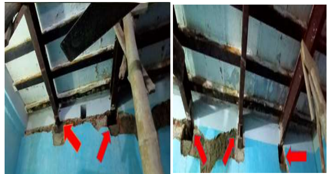
Figure – 7: Supporting the old joist roof with I section joist
