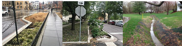
(a) Runoff from the vicinity flows into an adjacent bioswale (b) Swale drain
