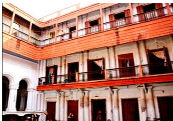
Fig.14: Straight Veranda on 1st floor
