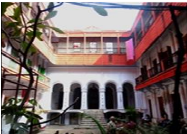
Fig. Existing courtyard, and thakur dalan of Mitra residence
