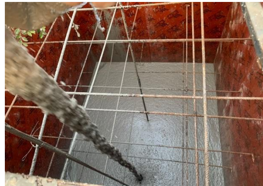
Figure 1 : Concreting of M60 TCC (Mock)
