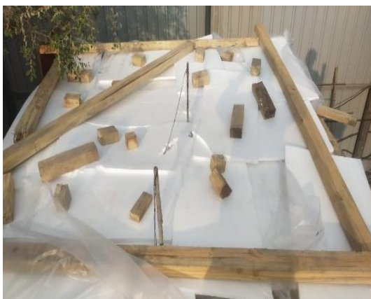
Figure 2: Insulation of Concrete (Mockup)
