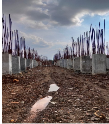
Figure 2. Construction of multi storey Buildings in progress
