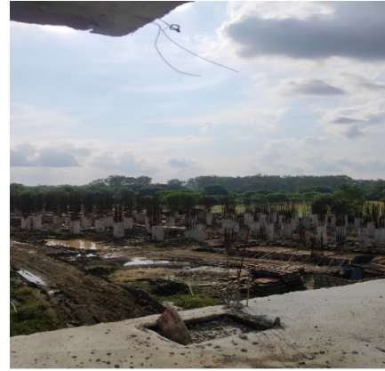
Figure 6. Top view of site under construction (SGS)
