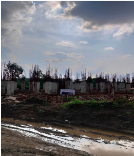
Figure 3. Construction of Duplexes in progress
